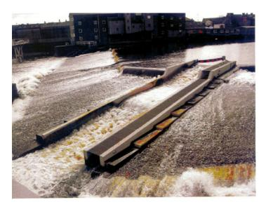
This gives some indication of the type of structure that is required. This weir has to be broken into with a section being removed. A concrete channel is then constructed with a series of baffles. The baffles slow down the water making it passable to fish.
